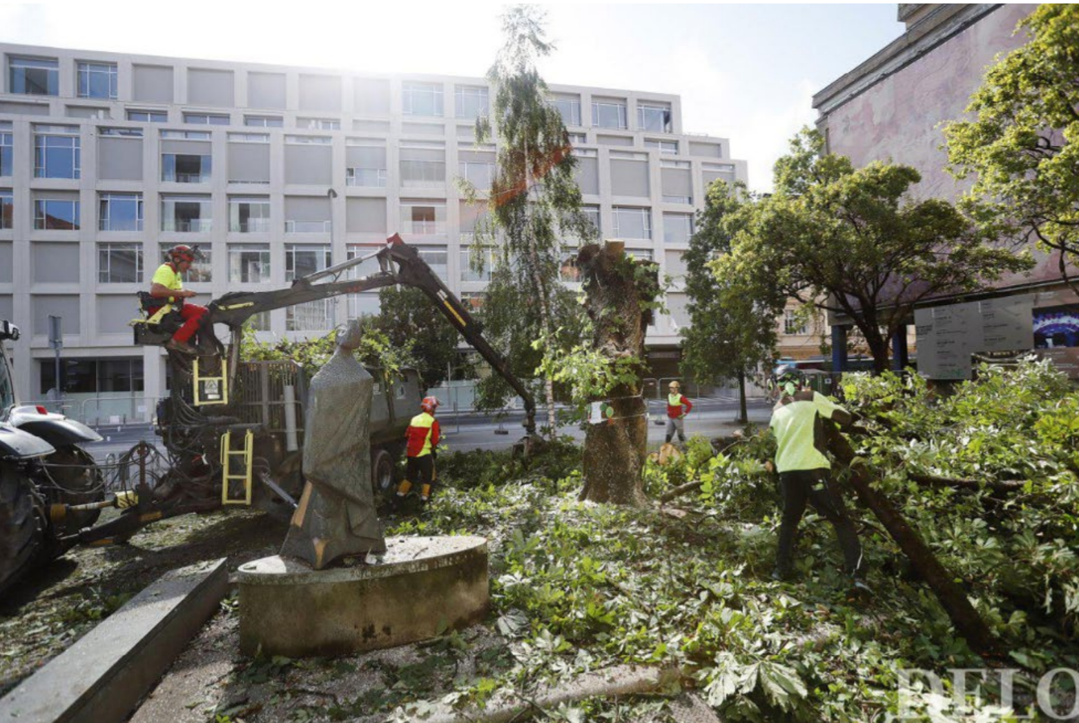
Cutting down monumental chesnut tree, Renovation of SNT Drama, 2023
